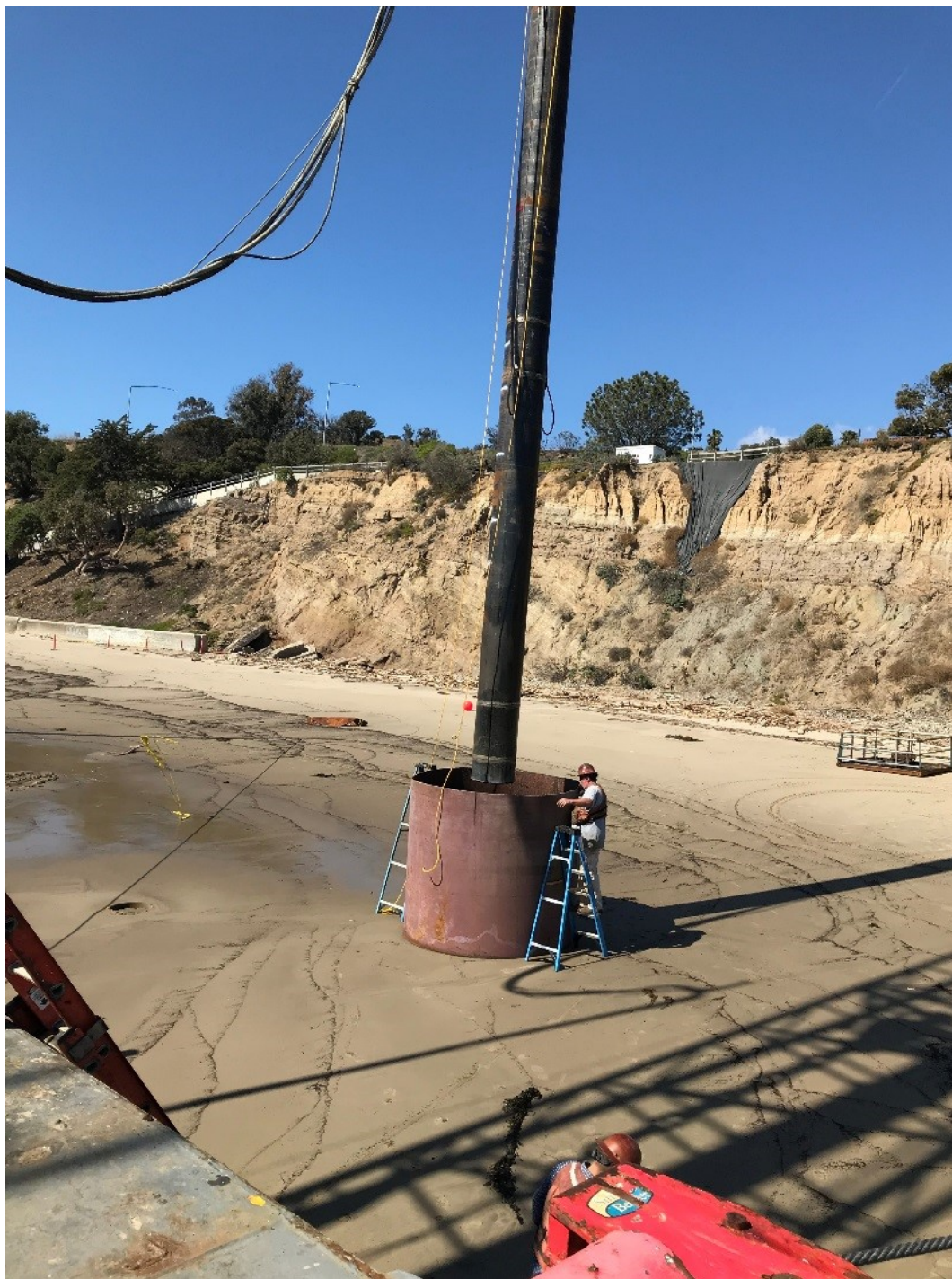
Figure 2-5. Installation of Steel Pipe Pile During Becker Well Abandonment
