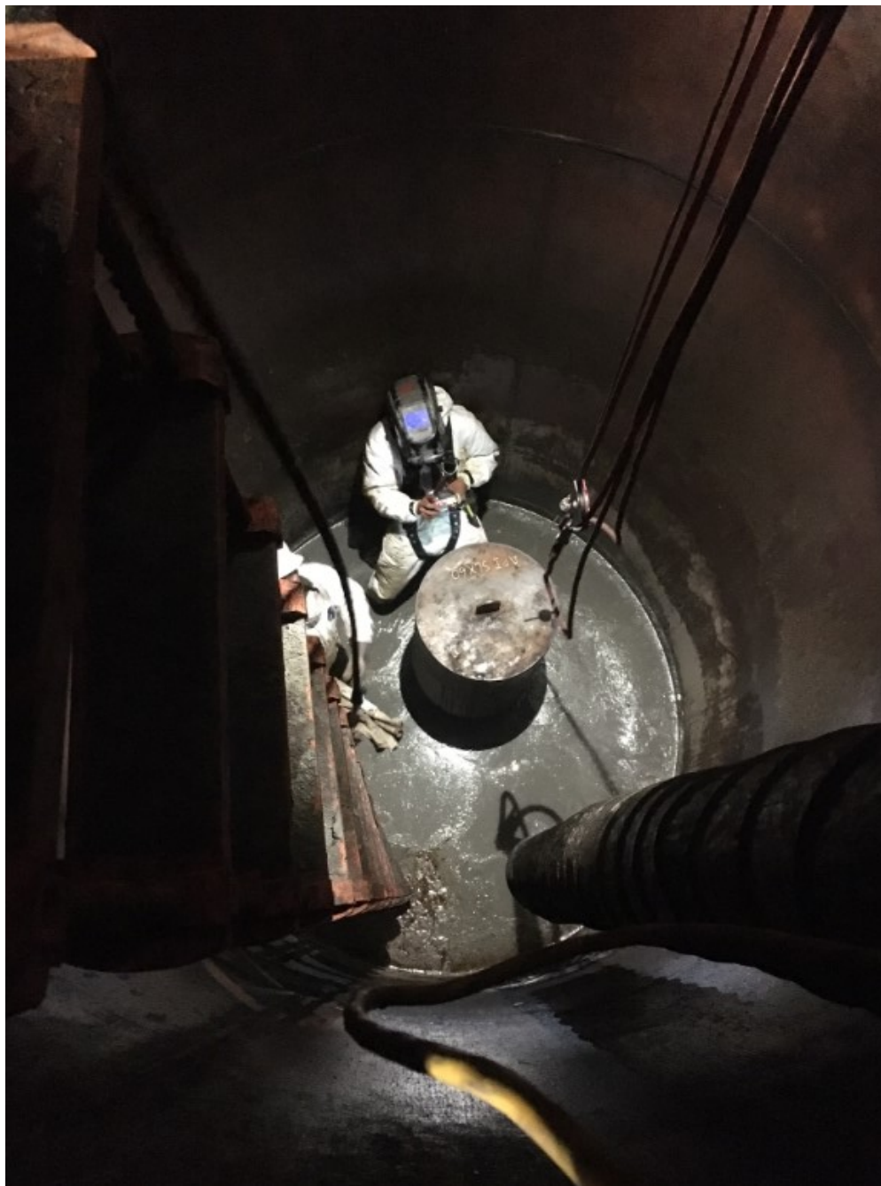
Figure 2-3. Welders Seal a Cap on the Becker Well Inside the Cofferdam
